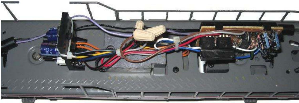
GP-20 before installation begins
